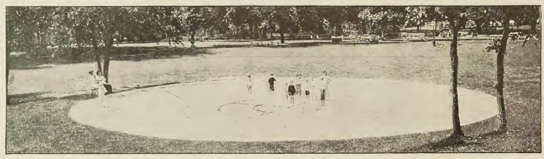
The thing that looks like a giant plate in the picture above is one of the wading-pools in the parks of Des Moines, Iowa. The water has been drained out to show the construction. The pool is made of concrete, and so designed that when filled the water gradually deepens toward the center, but is never deep enough to reach above a child's knees. Wading-pools will provide a nice, clean, safe and inexpensive amusement for the children in your town.
